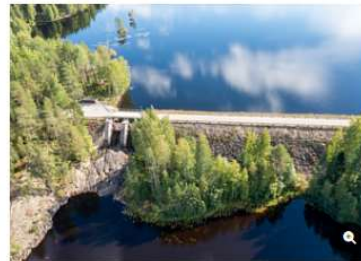
Hydropower dam that will be removed in Finland © Niko Jokinen
